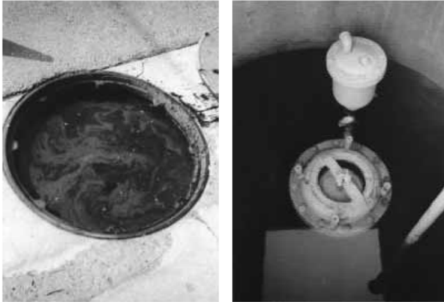
Figure 1. Submerged Air Valve Vault [LeChevallier]
