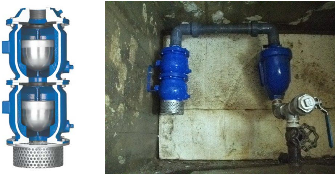
FIGURE 4. Typical ASSE 1063 Inflow Preventer Installation
