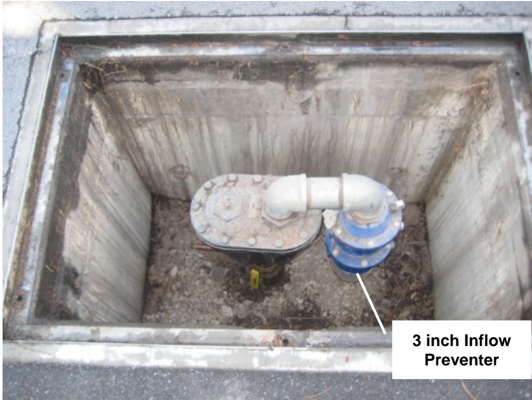
Figure 6. Air Valve Vault, Foster City, CA
