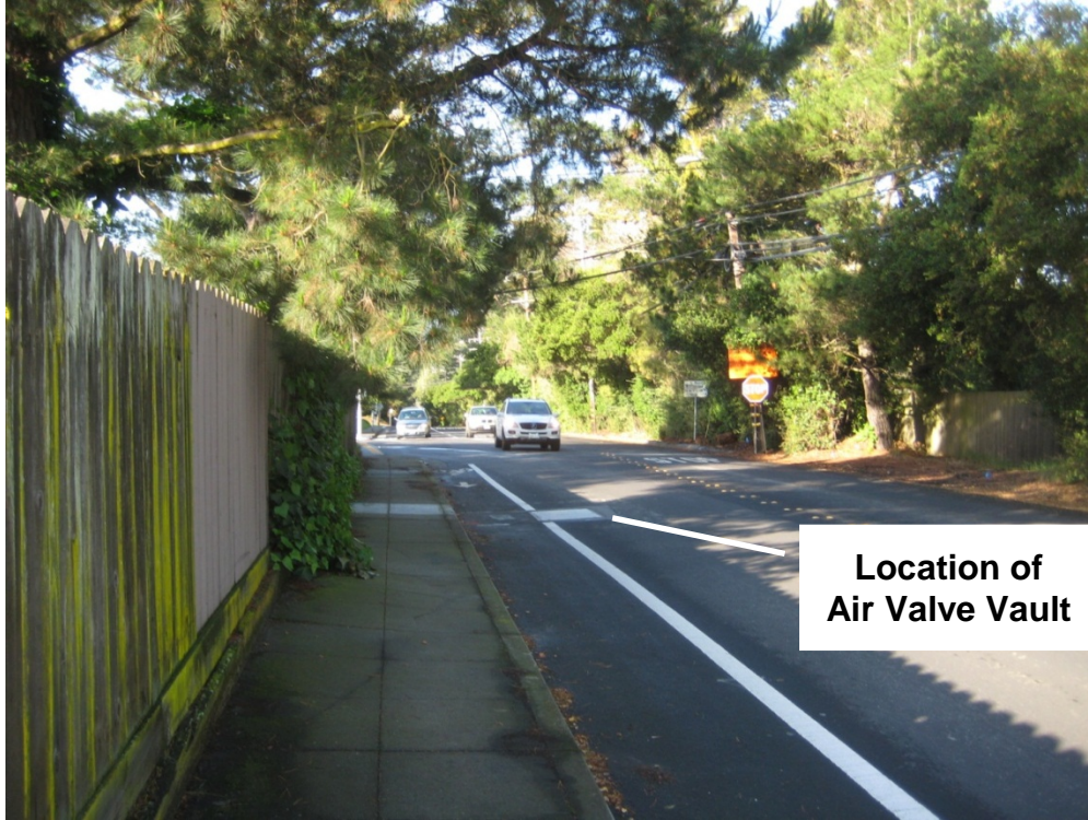
FIGURE 5. Water Pipeline in Foster City, CA
