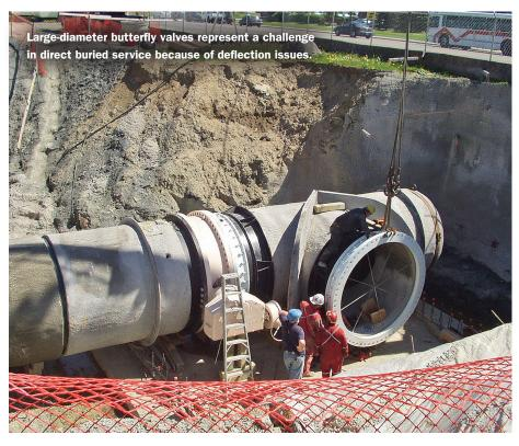
of external loads. With a large-diameter pipeline, this variance can represent several inches of vertical deflection. When the pipe and the valve are flanged together belowground, pipe deflections are transmitted to the valve and can be detrimental to the valve's integrity. The adjacent pipe connections must be supported and stiffened to eliminate the transfer of pipe loads to the valve. Where practical, the valves should be located in vaults.
