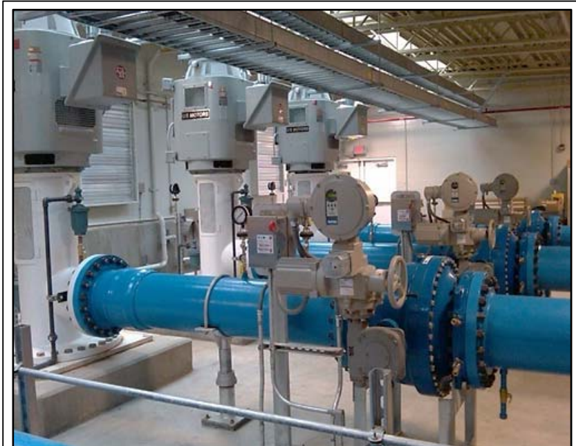
Figure 1 – Ener•G® Ball Valves at ECCV Treatment Plant
