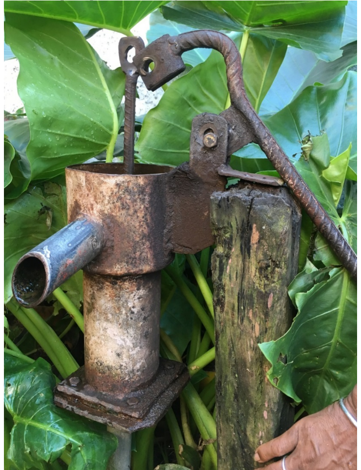
Another pump that is being rehabilitated
