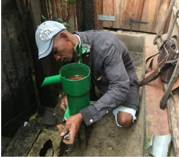
Nary working on pump
