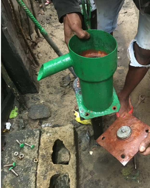
New lead-less parts being installed into the pump by local manufacturer.
