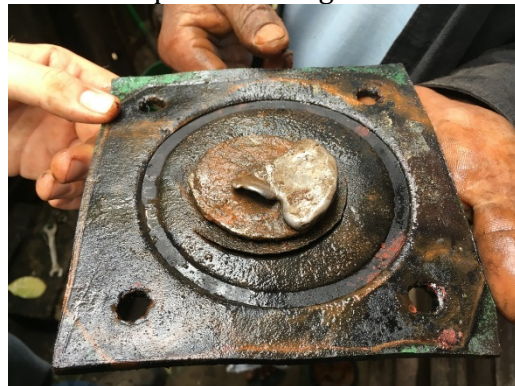
Example of lead weight used for check valve that was replaced during the intervention.
